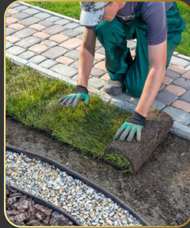
LANDSCAPE AND ASPHALT
